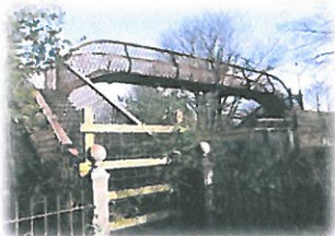
Photos of St. Mary's bridge and Upper Forge bridge.
