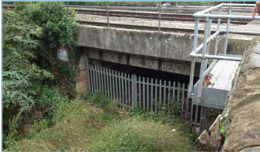
Figure 7.5 Current condition of the underpass on Station Road
