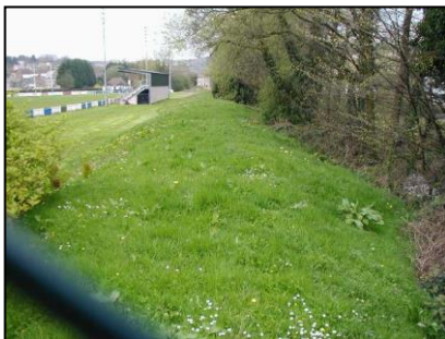
Figure 2 – Lydney 100yr Flood Embankment
