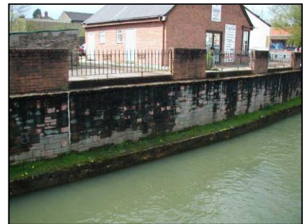
Figure 1 – Lydney 100yr Floodwall
